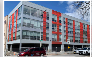
Corbett Corner, located at 444 E. Genesee Street, introduced 24 new affordable apartments in April 2022.
